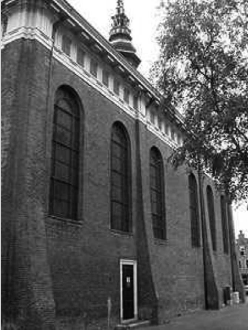
Figure 8: Nieuwe Kerk, Haarlem, south exterior wall
