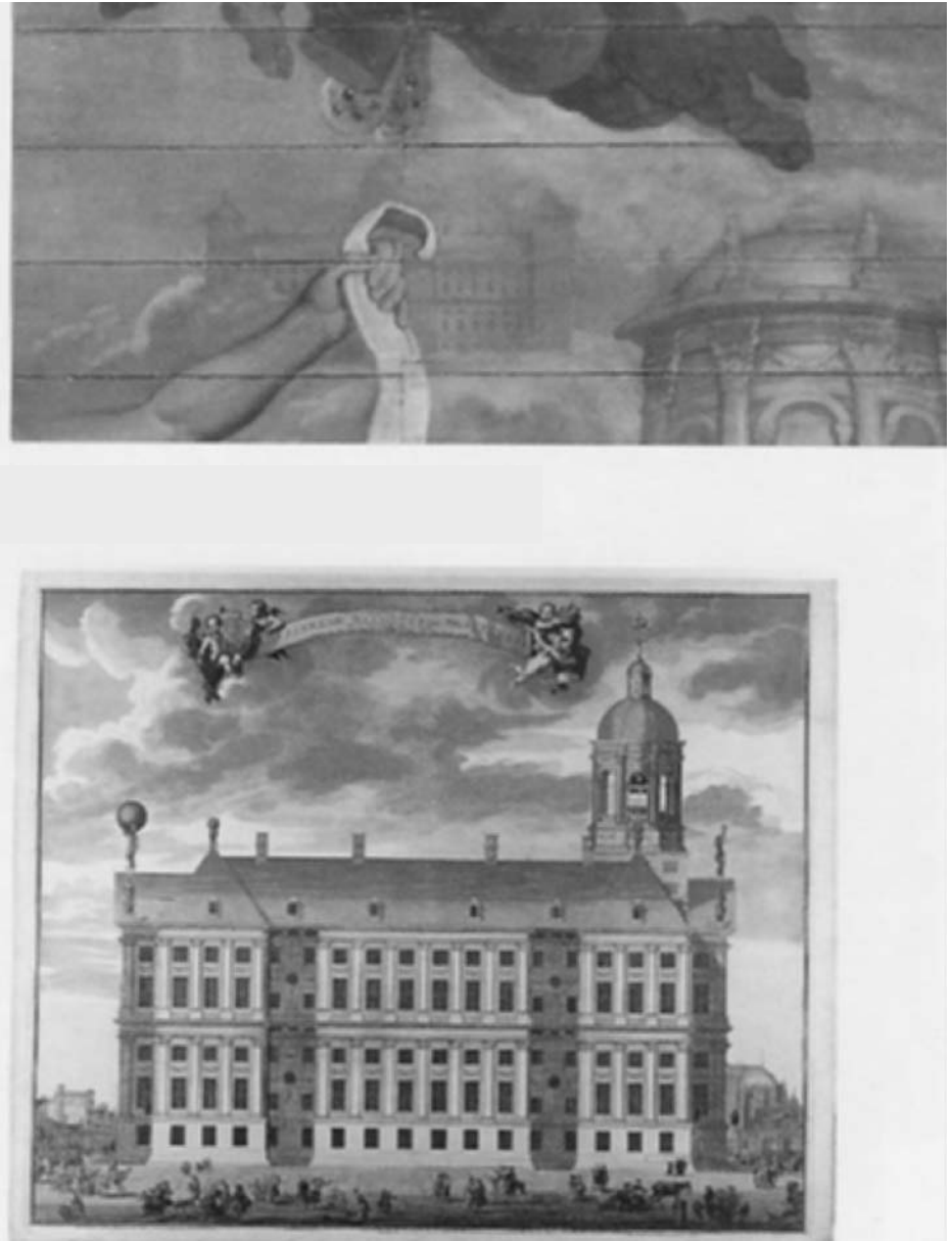
Figure 26: Detail of fig. 25 (above) compared to side elevation of the south side of the town hall of Amsterdam, published by Johannes Covens and Cornelis Mortier. (From article by Eymert-Jan Goossens in catalogue of Jacob van Campen exhibition, Amsterdam [Koninklijk Paleis] 1995, p. 215.)
