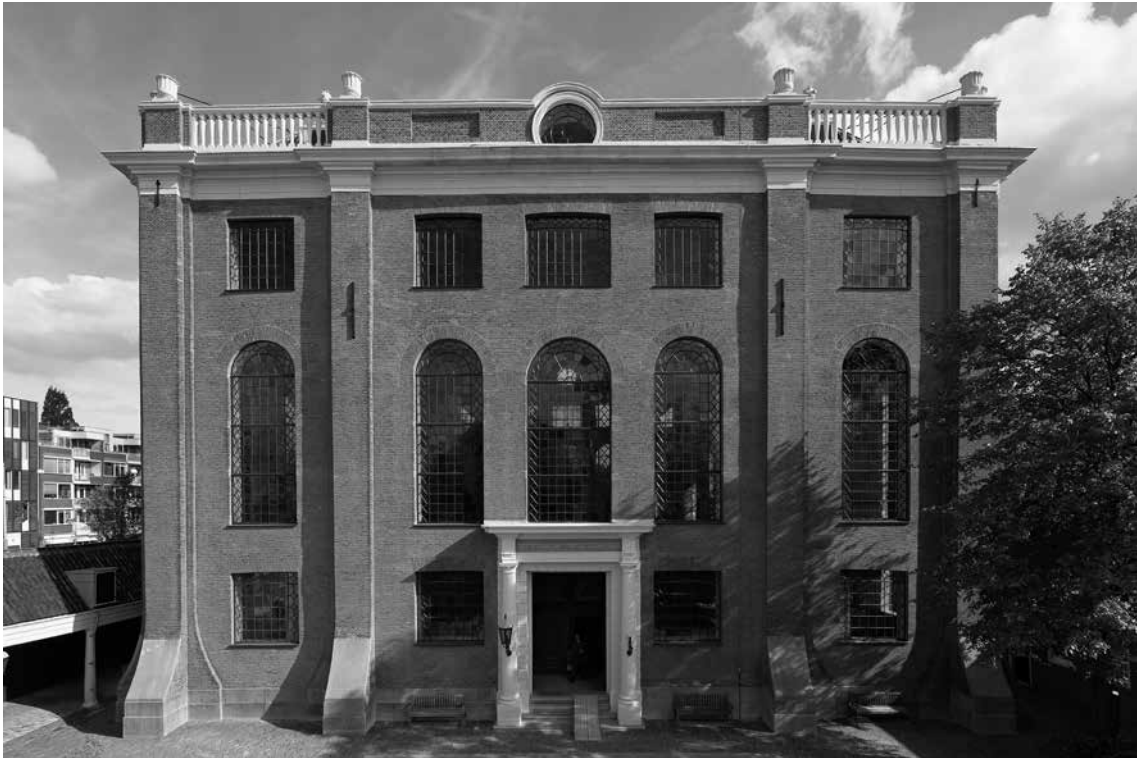
3. The exterior of the Portuguese Synagogue. (Photo: Dutch Cultural Heritage Agency)
